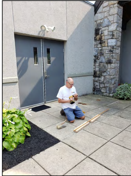
Mike Freshwater, working on the doors.
