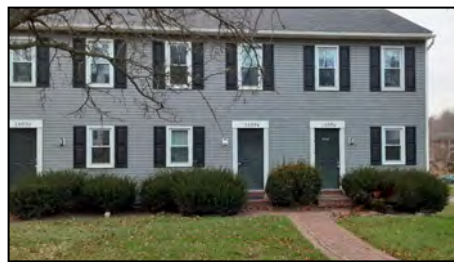
1609A Chadwick Circle, Lancaster, PA
