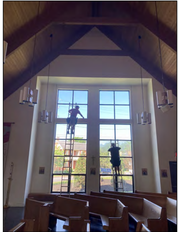
Washing the windows in preparation for the stained glass.
