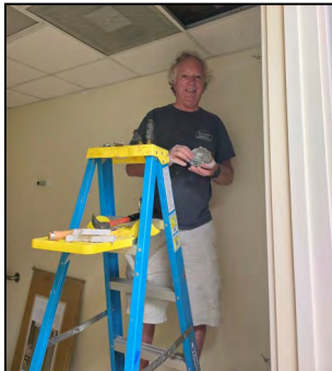
Bob Mutari working on electrical
